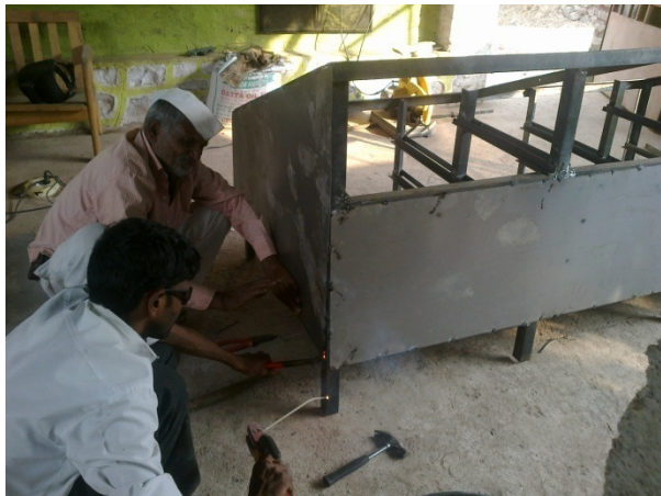
Bablu welding the tin sheet to metal frame of solar dryer
