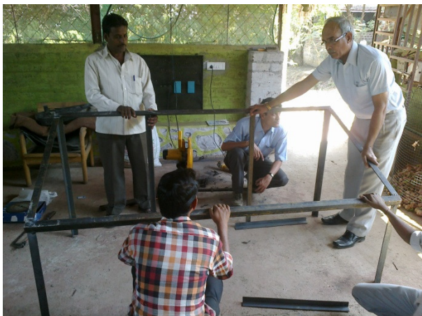
Welding the frame of the solar dryer at the Gorus workshop
